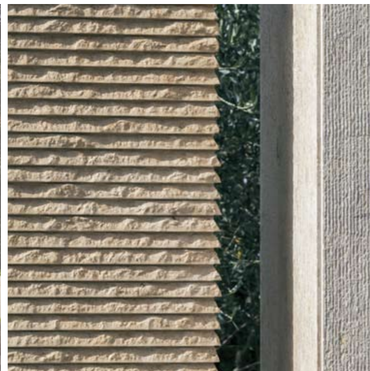
from above to below, from left to right: exterior view, view from the street, detail façade from stone and plaster
