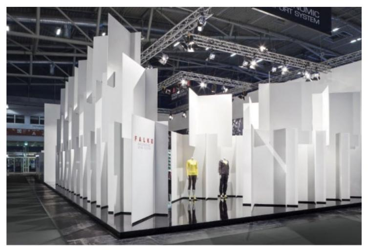
Wall panels with slits slot into one another to form the framework for the modular wall system. The structure is held together by its own weight, and even the taller walls can be put together without tools or any additional fasteners.
